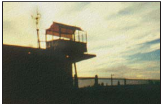
FIGURE 11-1 West Yellowstone Temporary Tower, 1988
