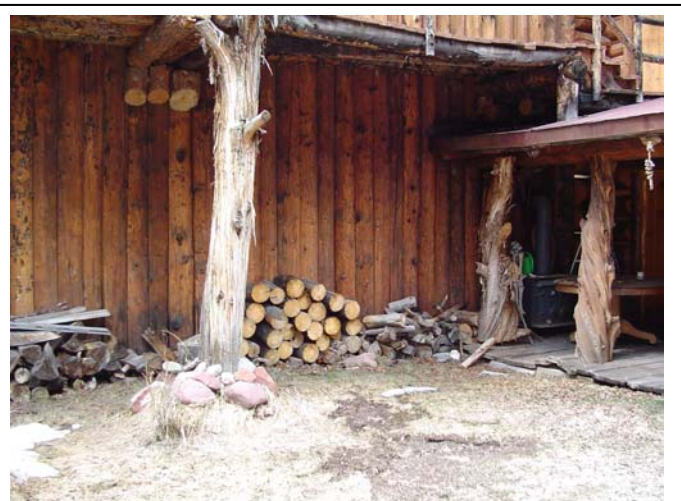
Do not store flammable fuels near walls, or under walkways.
