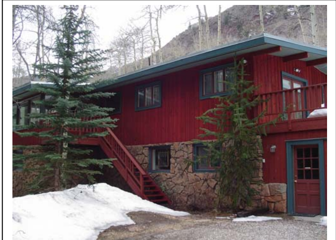
Flammable bristlecone pine underneath eaves is very hazardous, and should be removed.
