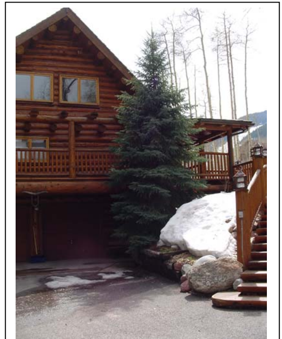
Consider removal of tree from adjacent to house, or ensure no litter or flammable material is below the tree. Limb tree up to 10'.
