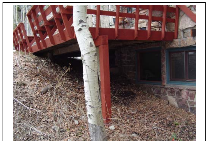
Remove all flammable materials from under porch, and enclose with mesh or solid walls
