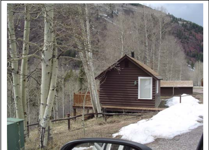
Remove vegetation from below porches, and keep grass mowed to less than 6” within 20’ of porches. Enclose deck that meets the ground at right side of cabin
