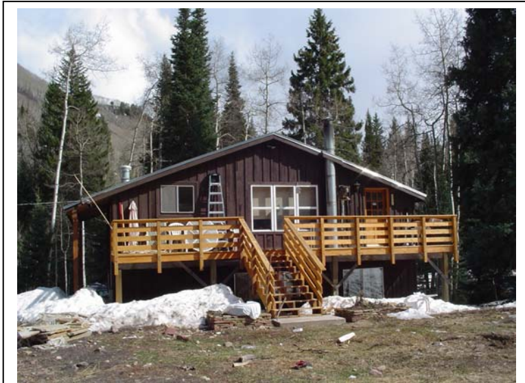
This duplex has mostly adequate defensible space, but needs some clean up of receptive materials immediately around the house.
