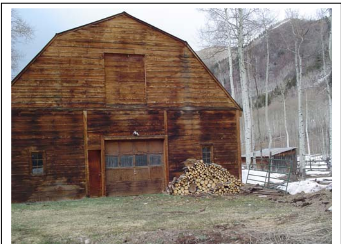
Move woodpiles and other flammable materials 30’ away from structures during the summer and fall months.
