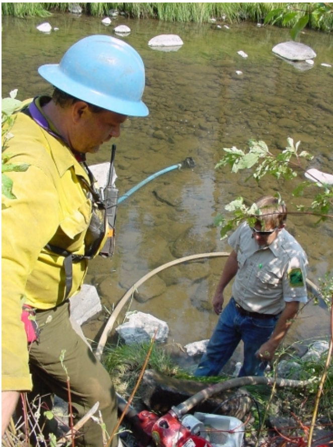
Figure 3—Pump intake screen submerged at the appropriate depth with clearance between the screen and any obstacles.
