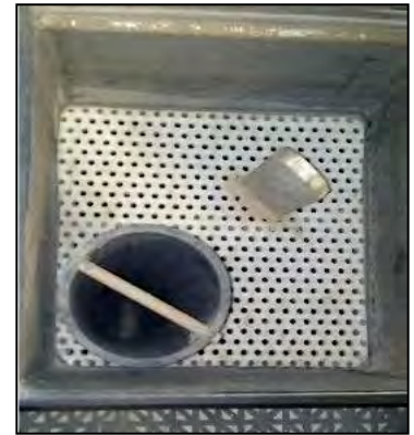
Tank Strainer Screen
