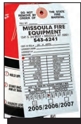
Figure 36—A fire extinguisher inspection tag.
