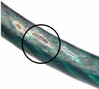
Figure 5. Damaged plastic coated wire rope.
