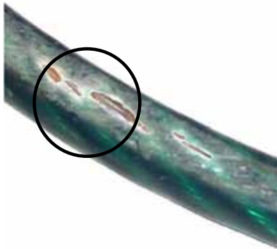
Figure 6. Damaged plastic coated wire rope.
