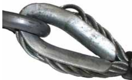
Figure 8. Deformed Thimble and Hook.
