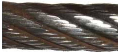
Figure 7. Abrasion and Corrosion extends through plastic coating to wire rope.
